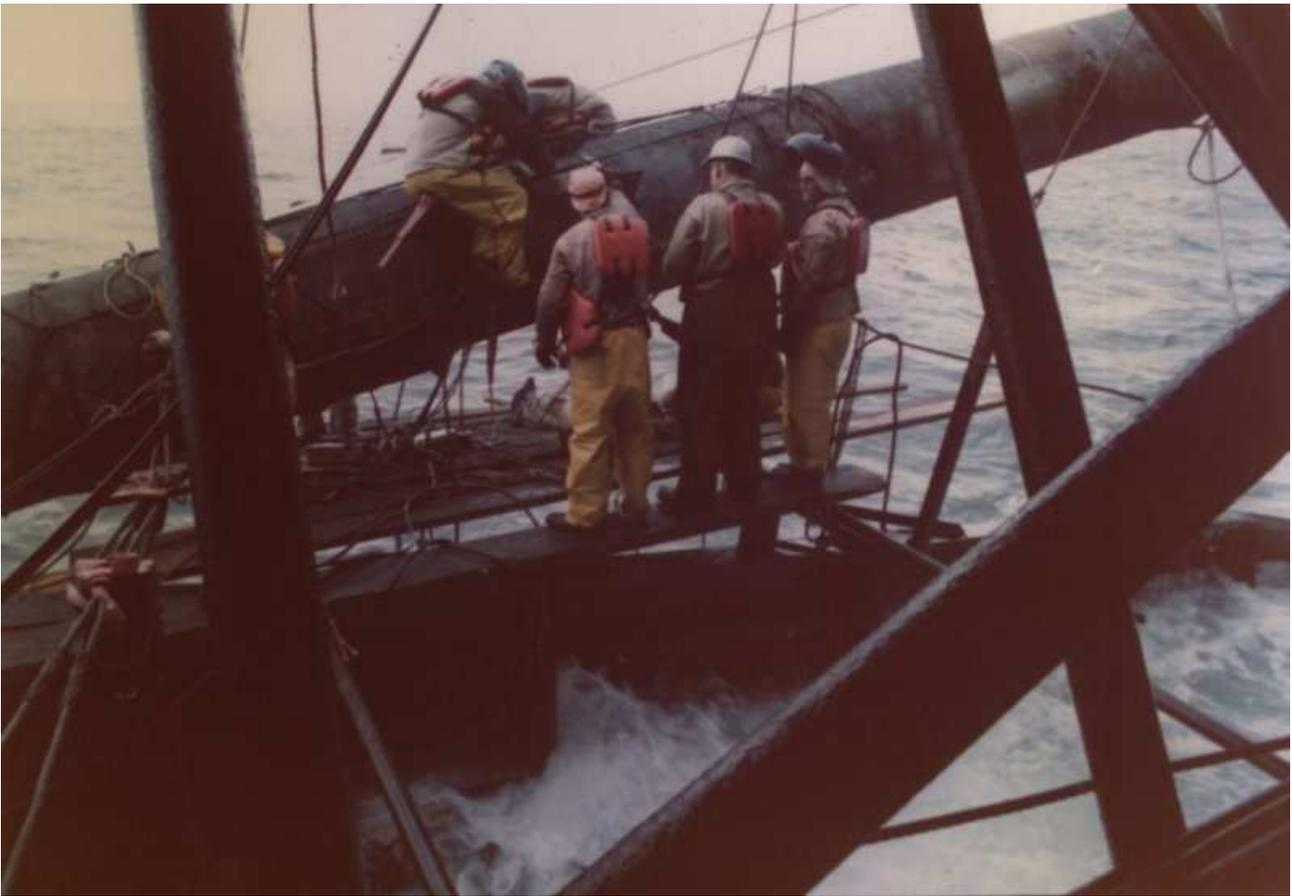
The deck crew has aligned the two pieces and the welders are now doing a full weld to the pipe. After X-raying the weld the steel pipe will receive a 3" layer of Tar to protect the steel from rusting.
